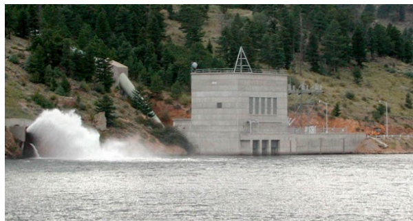
Mary's Lake Power Plant
