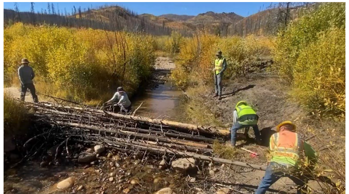
Crews placed post-assisted log structures (PALS) on Forest Service land within the burn area of the 2020 East Troublesome Fire.
